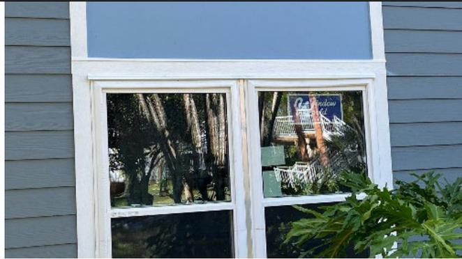
Side-by-side window, with the central aluminum mull bar without the clipped snap trim finishing
