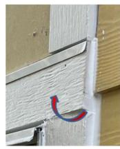
The top trim removal can damage the metal flashing above it, be careful.
